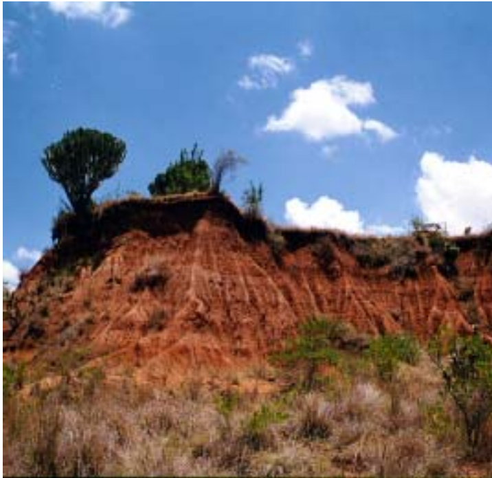
Figure 1.13: Gully erosion at Ol Donyo farm. Image by B. Sturm.
